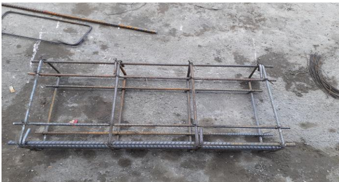
e) Steel Reinforcement
