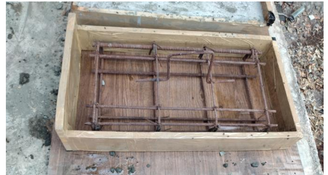
j) Wooden box for casting deep Beam
