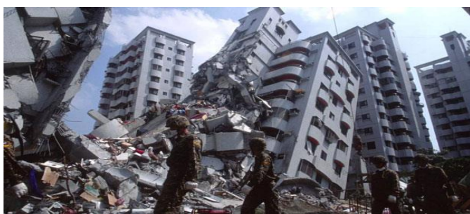
Fig -1 Damages to the building during earthquake
