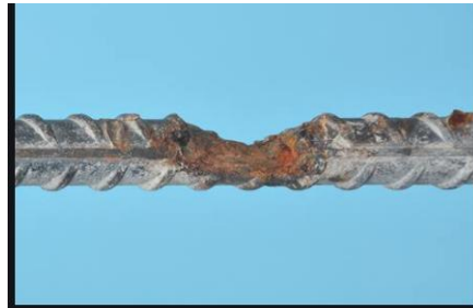
Fig-2: Pitting corrosion
