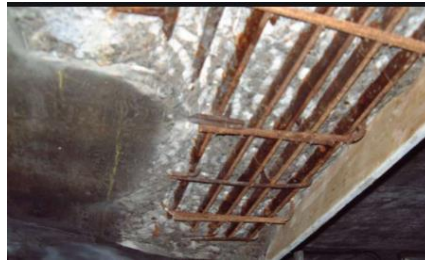
Fig-1: Durability issue due to carbonation
