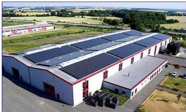
Fig 4: Solar System for Factory.
