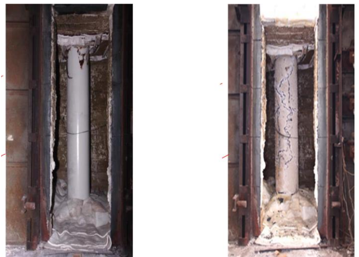
Figure (4) Test of IFC protected specimen before and after testing
