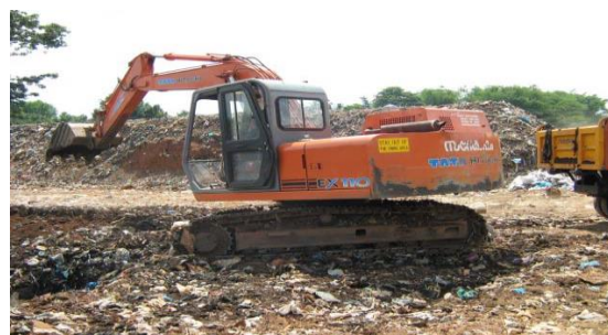
Fig-4: Removal of waste in segment B
