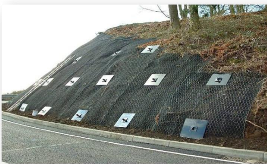
Figure: Typical Soil Nailing
