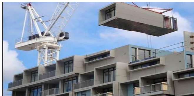
Fig 1: 3-D Volumetric Construction
