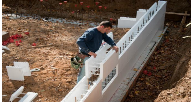
Fig 8: Insulating Concrete Formwork (ICF) Technique
