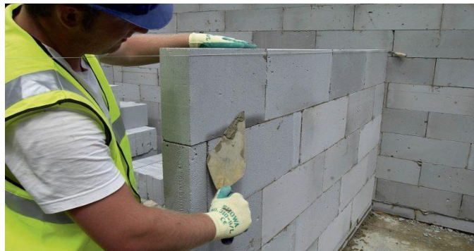
Fig 7: Thin-Joint Masonry Technique
