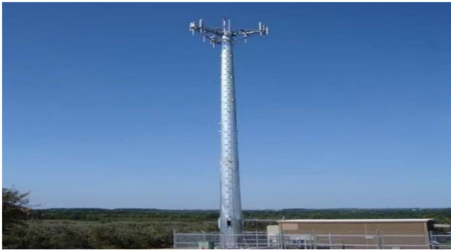
Fig:3- Monopole Tower
