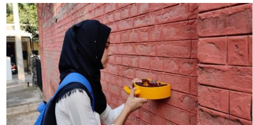
Fig 2 . Conducting Non-destructive testing
