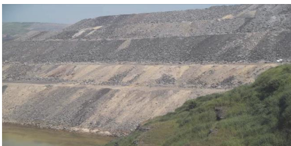
Fig 2: Decks with Fly ash as admixture in overburden material after compaction
