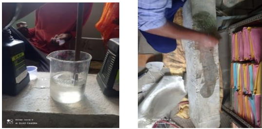
Fig -3: Application of epoxy and hardener on the beam
