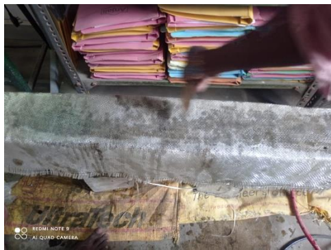
Fig -4: Fixing of GFRP sheets on the beam
