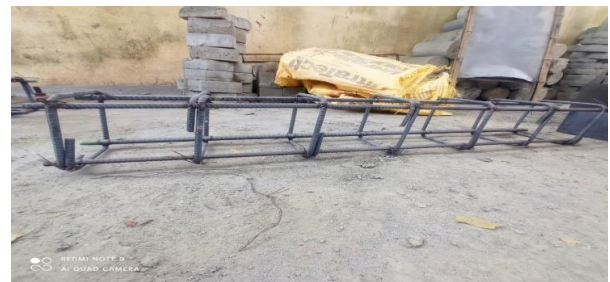
Fig -1: Reinforcement Detailing of Beam
