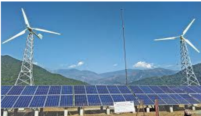
Fig -3: Hybrid Wind solar power plant installed at the HariharpurGadi area
