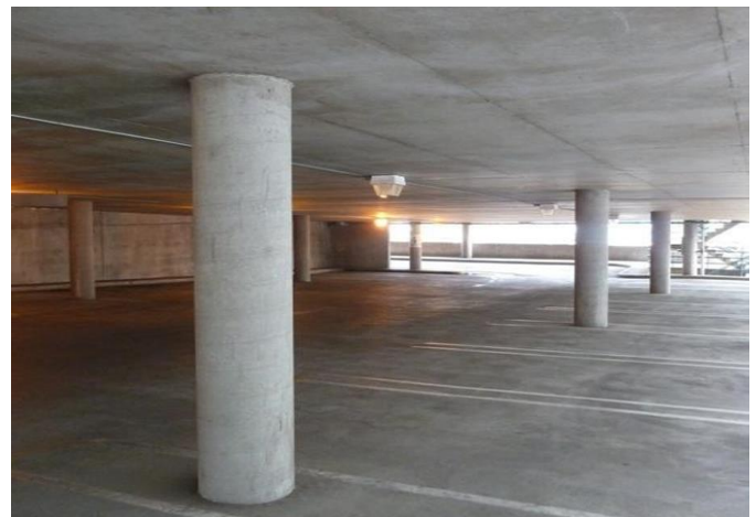
Fig 1. Typical flat slab construction
