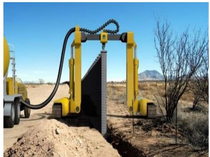
Fig -1: New Technology in Construction
