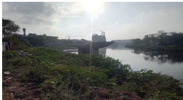
Fig 10: Construction work at place
