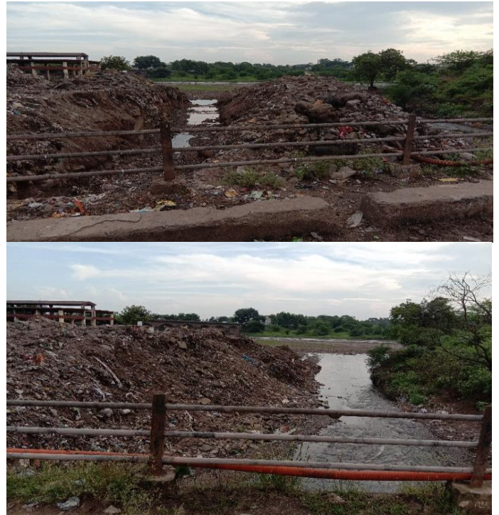
Fig.2. Showing landfill site at bank of Bhima River after site excavation
