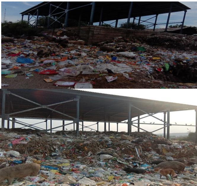
Fig.1. Showing landfill site at bank of Bhima River before site excavation
