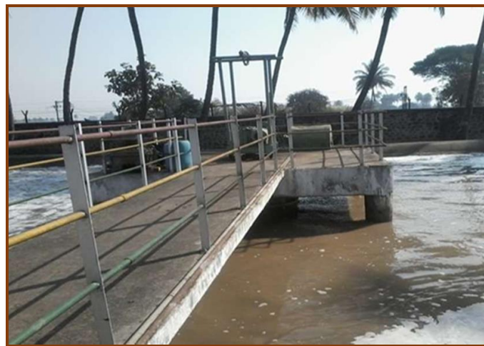
Fig -2: Effluent Treatment Plant
