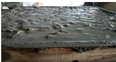
Casting of cement and wood pieces
