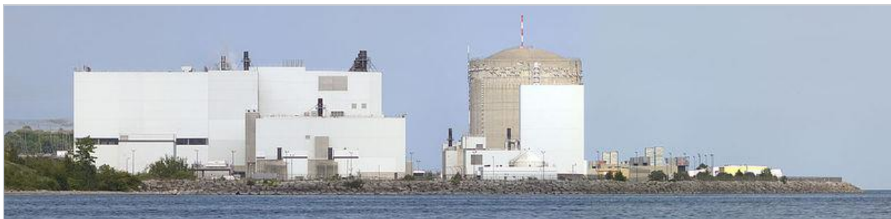
Figure 1. The Darlington nuclear power plant in Ontario produces power from four 878 MW CANDU reactors.
