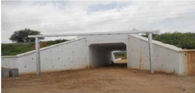
Fig-3: Road under bridge
