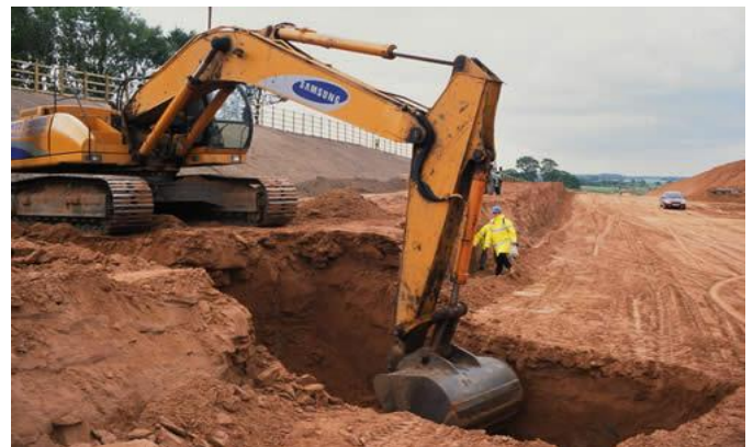
Fig-5: Excavation process
