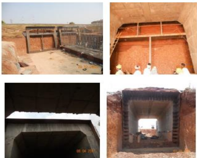
Fig-7: Casting of RCC box segments
