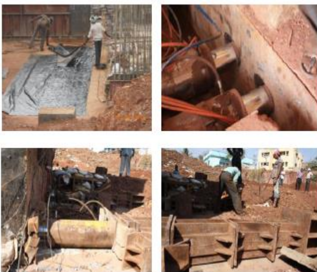
Fig-8: Pushing box segments using hydraulic jack
