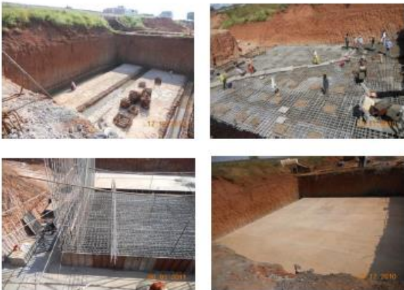
Fig-6: Construction of thrust bed
