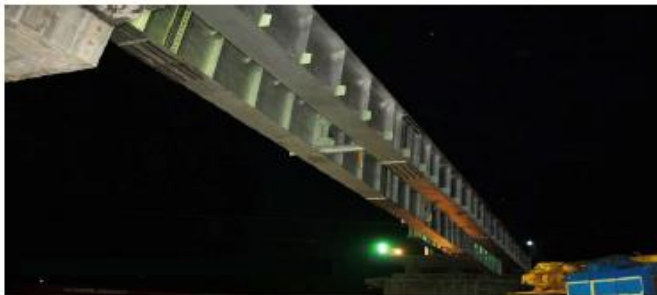
Fig-4: Road over bridges
