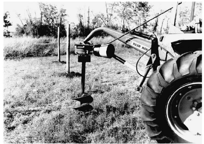
Fig 2.4 Tractor Driven Post-Hole Driller
