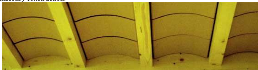
Fig-13: Exposed terracotta ceiling blocks providing thermal mass to timber frame construction
