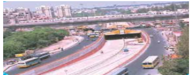
Figure 6. Level Traffic Interchange Integrating Road and Metro
