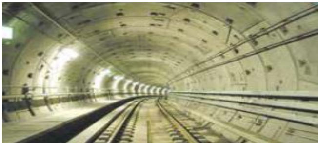
Figure 4. Underground Metro Tunnel Using Precast Segments
