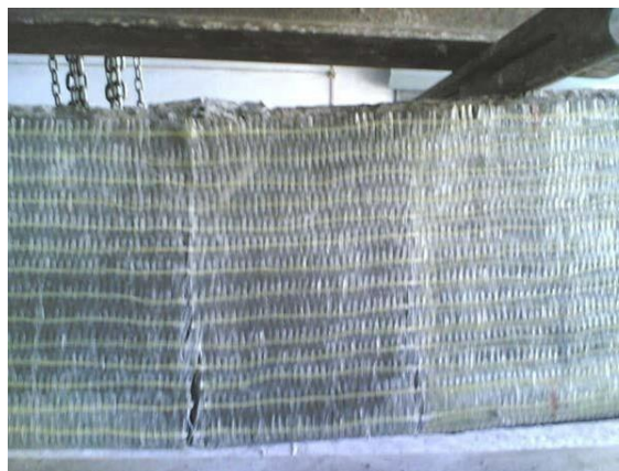
Fig-1 Failure of Beam Retrofitted with GFRP Jacket with fibers at zero Degree to The Longitudinal Axis of Beam
