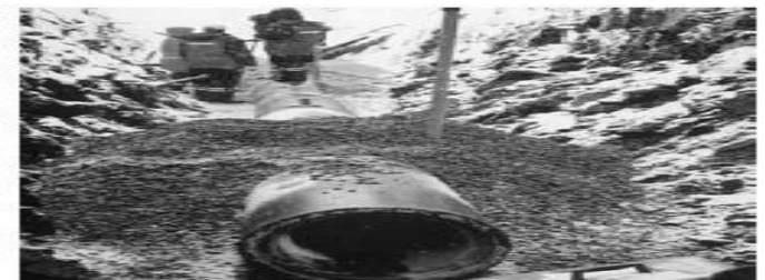
Figure 7. Recycled Aggregate as Backfill Materials
