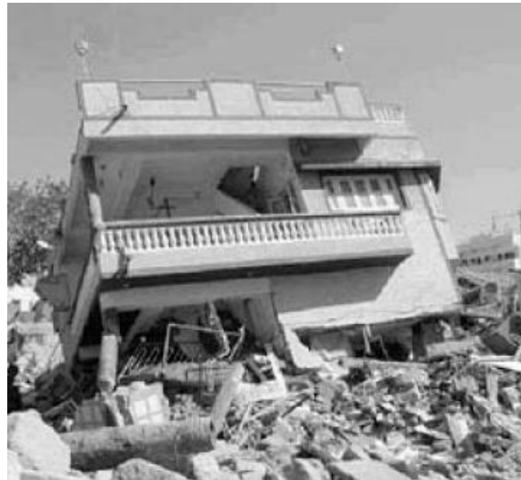
Figure 1. Soft Storey Failure in Bhuj
