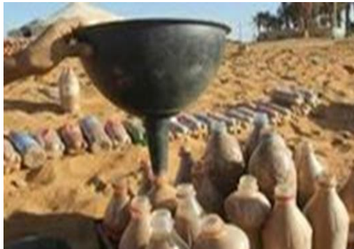
Fig 8. Filling the bottles with sand
