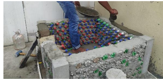
Fig 11. Construction of pet plastic bottle room
