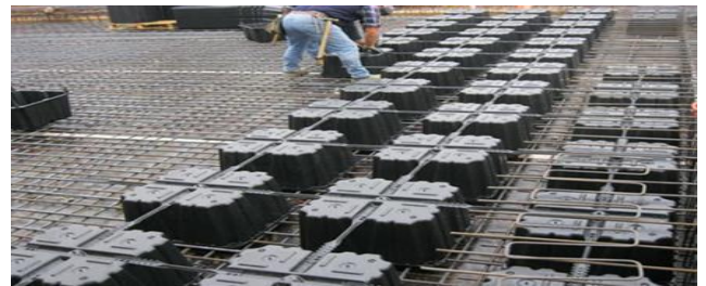
Fig 3. U-Boot technology in slabs
