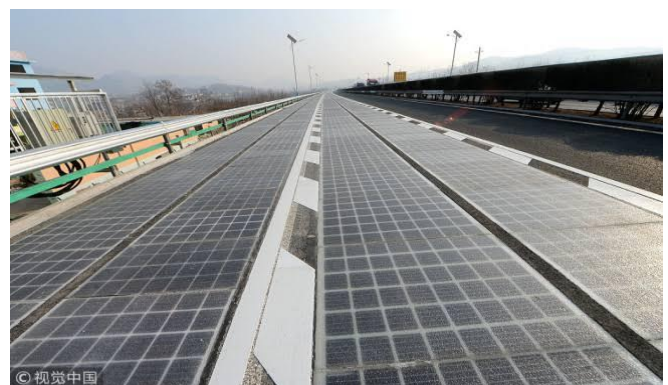
Figure 4.1 Shandong Project Solar Road
