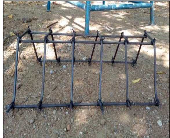
Fig-3.3a Trough shape reinforcement
