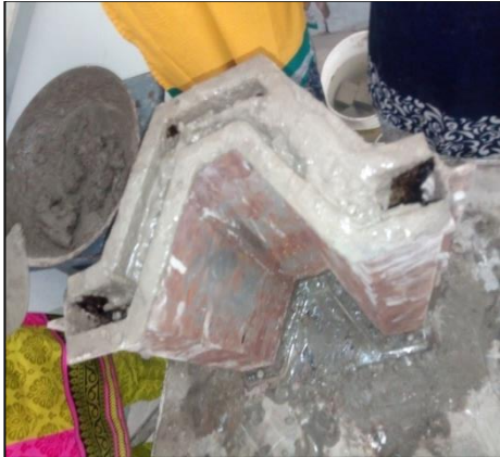
Fig-4.1 Placing of concrete
