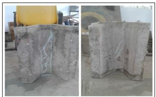
Fig-5a Tested Specimen showing crack details
