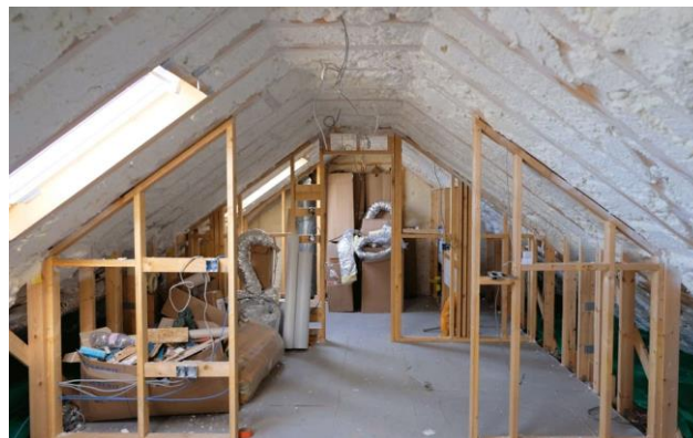
Fig. 5: Attic Insulation by Spray Foam
