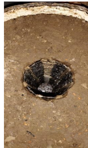
Fig-3.5.1: Stone column reinforced with geogrid
