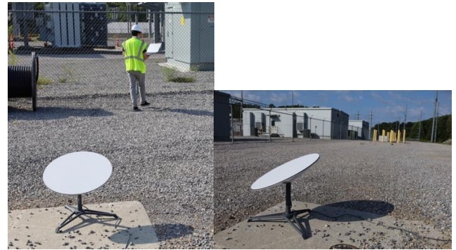
Fig. 8: Starlink transceiver deployed at utility substation.
