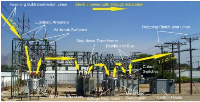
Fig. 5: Energy flow in a generic electrical substation.
