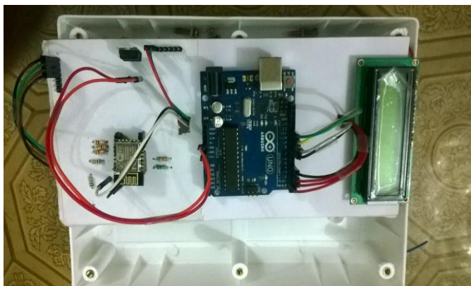
Fig -5: Smart Energy Meter
