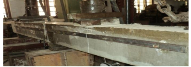
Figure 3.33 Strengthening and anchoring pattern of SB9
