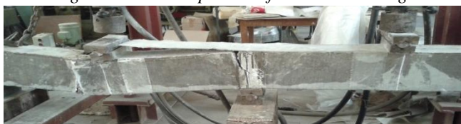
Figure 3.23 Failure of the beam by tensile rupture
