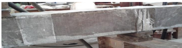
Figure 3.22 Crack pattern after initial loading
