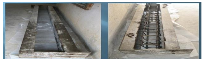
Figure 3.3 Steel Frames Used For Casting of Beam
