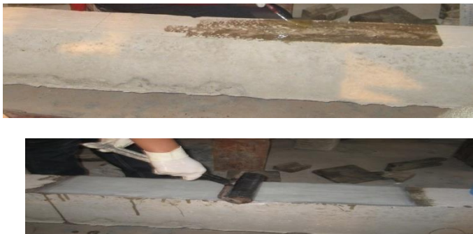
Figure 3.5 Roller used for the removal of air bubble
