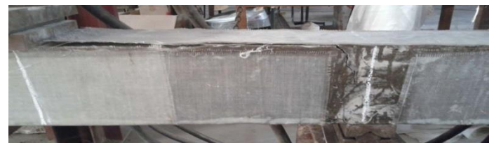
central support of the beam
