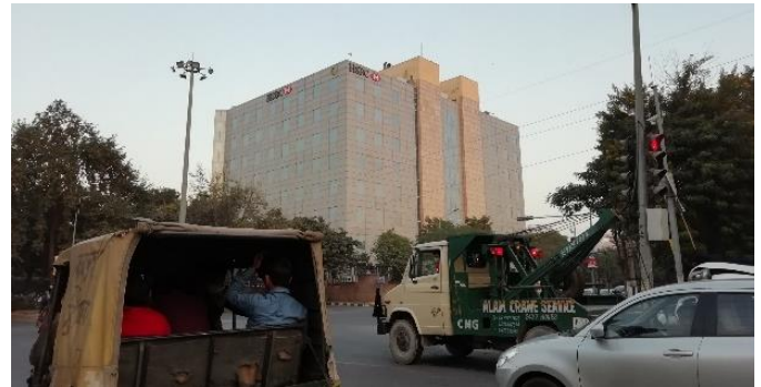
Fig -22: HSBC Building, Front
