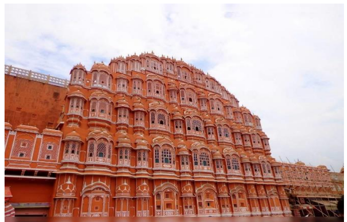
Fig -10: Hawa Mahal (Source: Pipralia, 2014)
