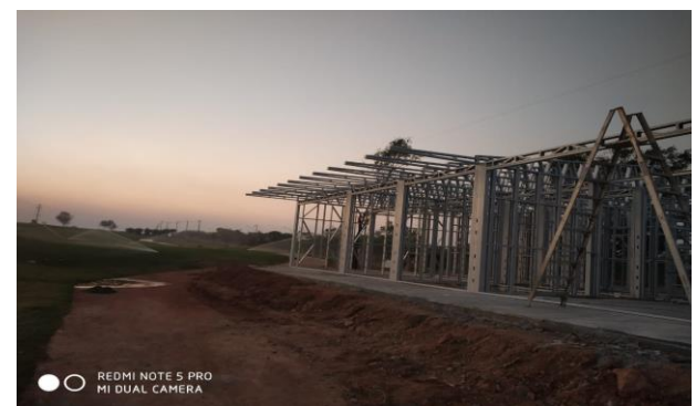
Fig -6: Actual construction site picture
