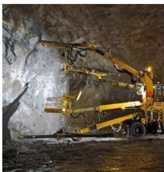
Fig -2: Drilling by drill jumbo
