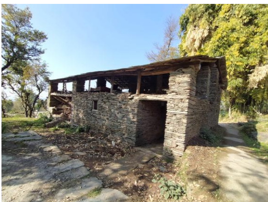
Fig- 7 Dry Stone Construction
