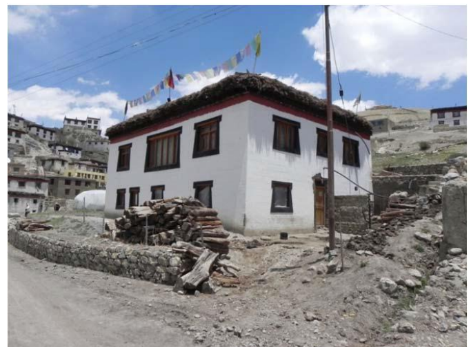
Fig - 5 Mud Construction in Alpine Zone
