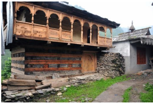
Fig 6 Kath Khuni Construction
