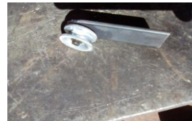
Figure 17. Pulley welded to the sill to pass the tensioned rope.
