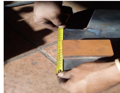
Figure 15. Placement of motor base.
