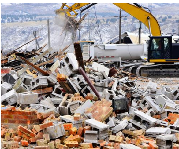
Fig -1: Building Demolition
