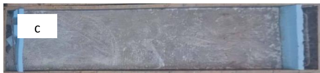
c) Painting the surface with epoxy resin (Epoxy-R)
