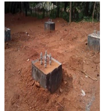
Fig -10: Backfilling
