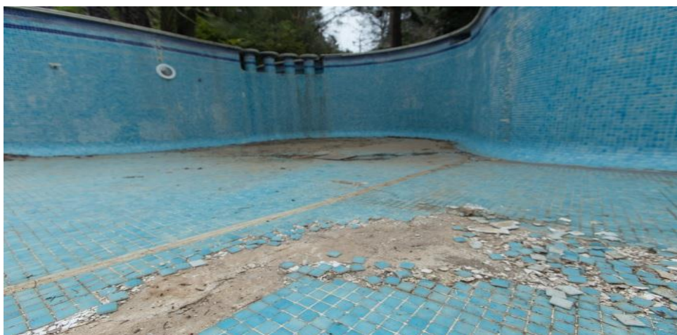
Fig 1.2 Earthquakes Impact In Pools Flooring
