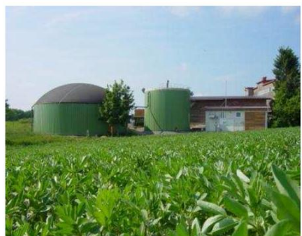
Fig -6: Vertical digester in Germany, processing pig and poultry manure and crop silage
