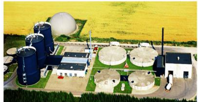
Fig -8: Picture of centralized co-digestion plant in Denmark (LEMVIG BIOGAS)
