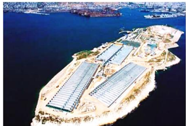
Fig -11: Waste water treatment plant in Psyttalia, Greece (FARNSWORTH 2004)
