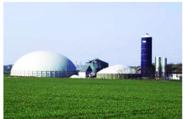
Fig -5: Picture of farm scale biogas plant in Denmark, co-digesting animal slurries and energy crops
