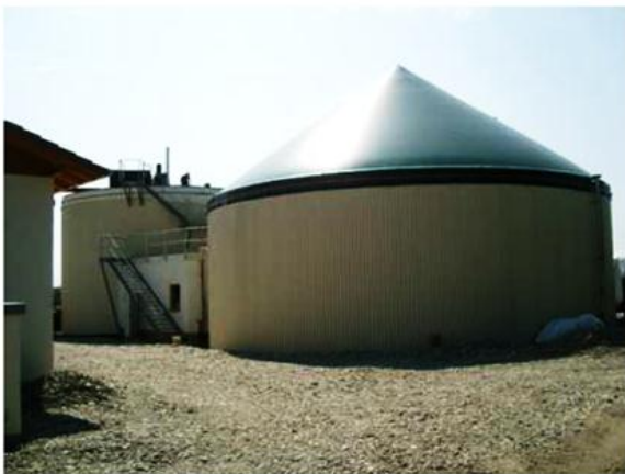
Fig -7: Vertical digester in Germany, built in 2005 for digestion of energy crops
