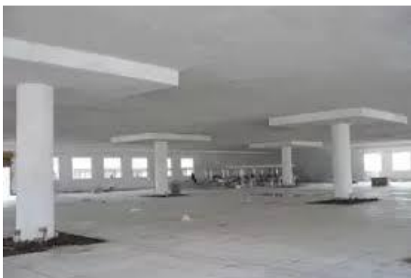
Fig -1: Reinforced Concrete Flat Slab
