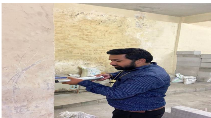
Picture 1: Rebound Hammer NDT Testing on Column
