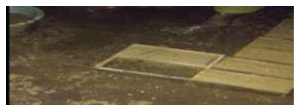
Fig-3 Hand moulding of bricks
