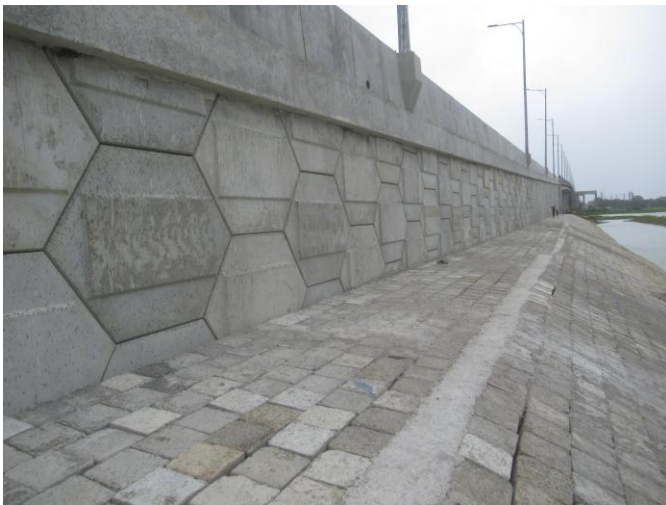
Fig -13: Photo of Nehemiah Wall at Embankment
