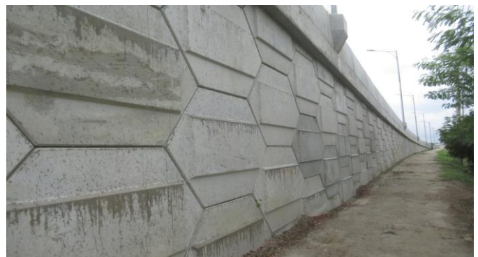
Fig -12: Photo of Nehemiah Wall at Approach Road
