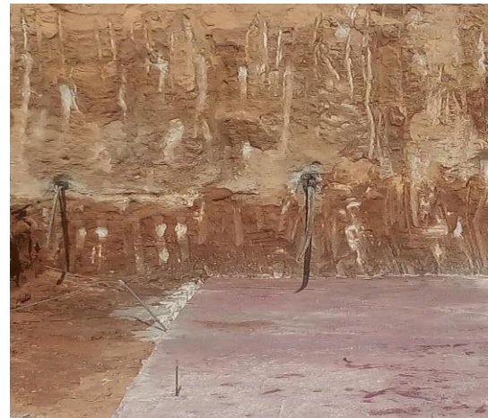
Fig 4.2 Anchor fabrication
